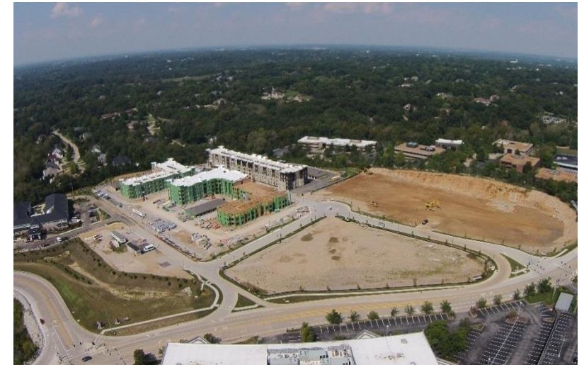
2016: New construction underway, major mixed-use development
