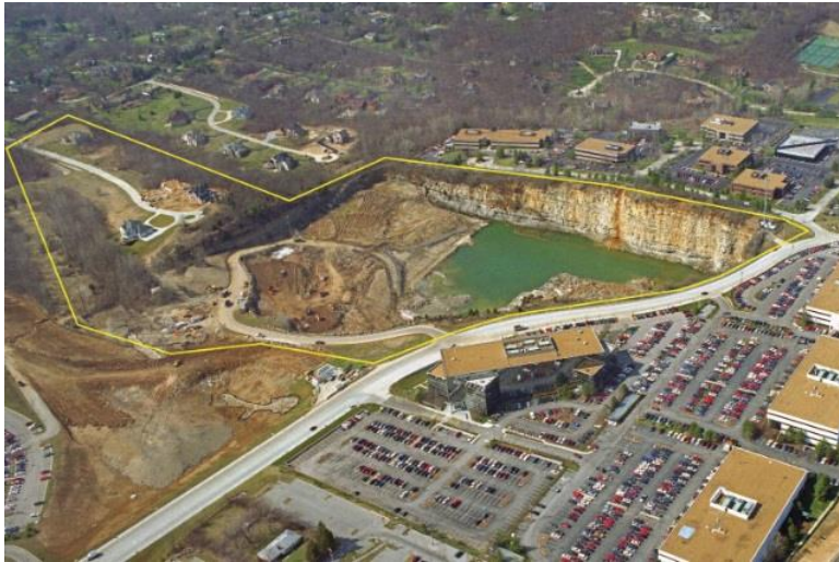
1994: 180 ft deep rock quarry, environmental hazard
