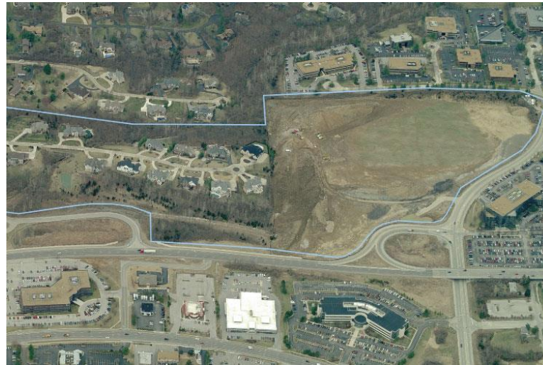
2014: CDC completes environmental restoration
