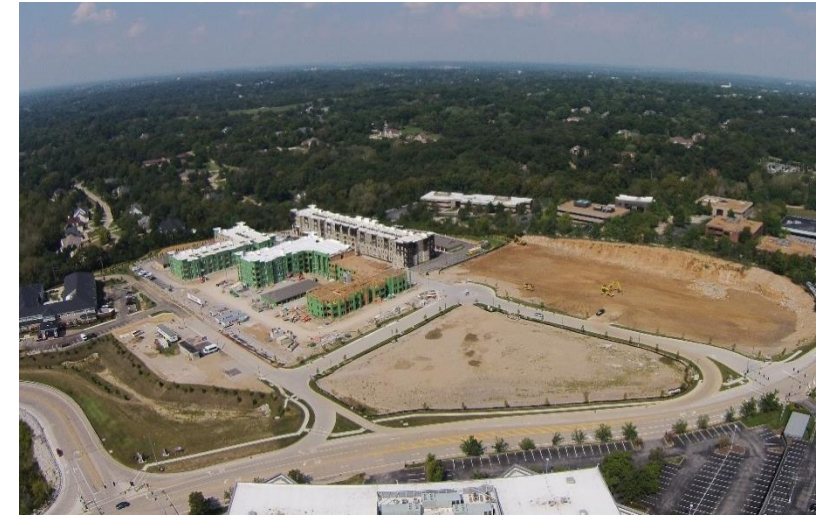
2016: New construction underway, major mixed-use development
